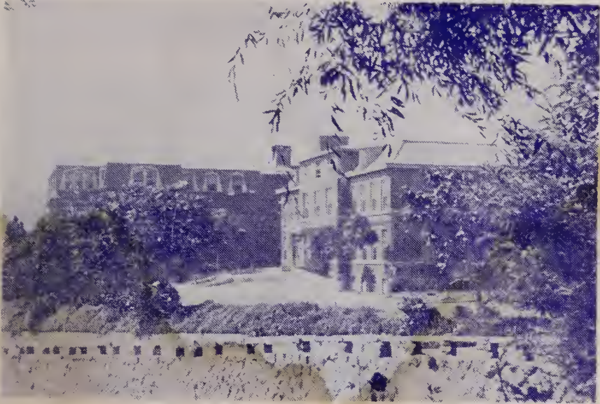
Out-patient Clinic (Rt.) and Main Hospital Building (Lt.)
